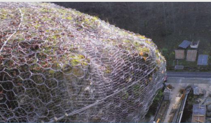
Heavy rock stabilization using Omega-Net.
