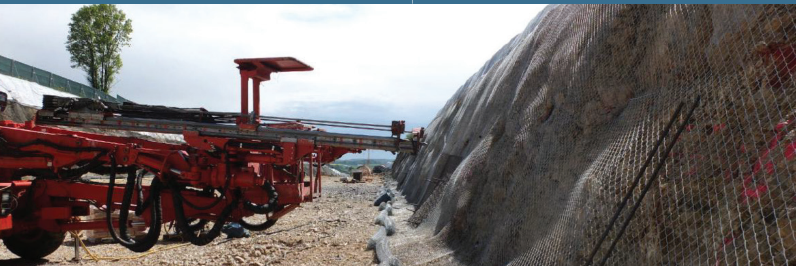
Slope stabilization using a combination of rectangular mesh and anchors.
