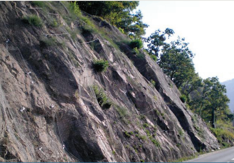
Hexagonal mesh can be used for slope retention systems where the forces are not high.
