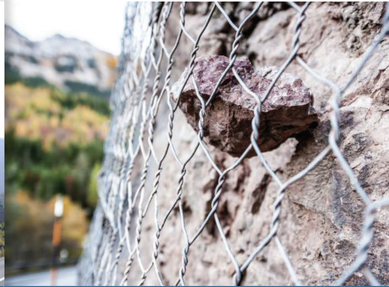
The thick, malleable wires used for hexagonal mesh, along with the twisted interlocking of the strands yields a flexible product with redundancies.
