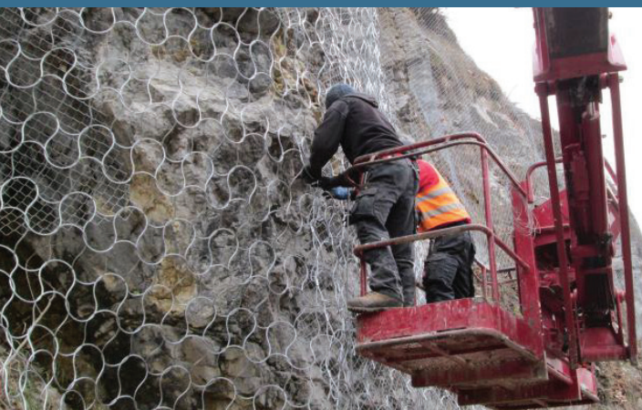
Installation of Omega-Net for slope stabilization.
