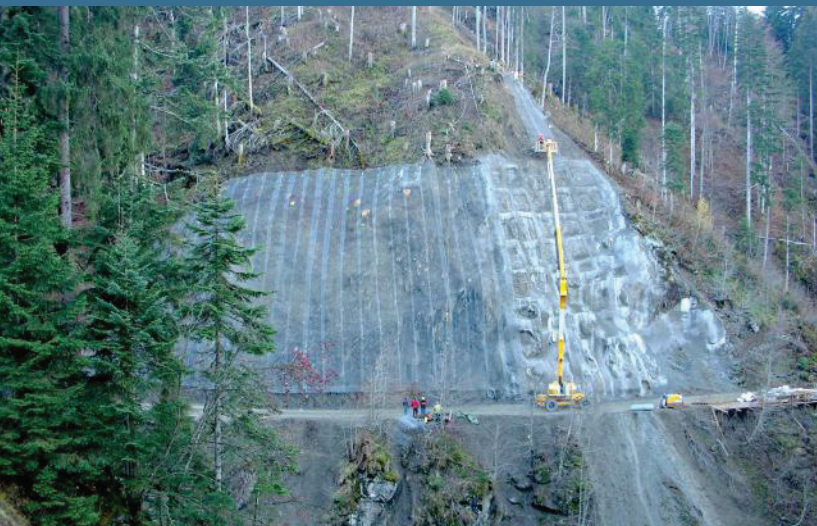
The light weight, long rolls make them ideal for covering large areas of slopes that are affected by unraveling and other mass wasting processes.
