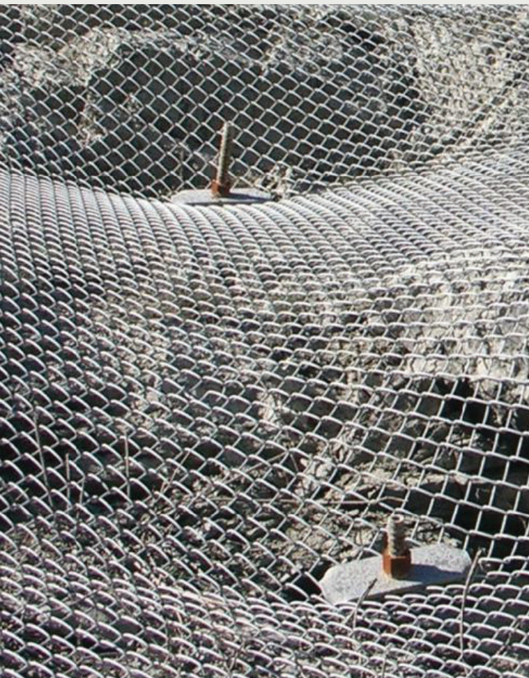
An example of interior anchors using a standard spike plate for the coupling. Anchor points are typically set in topographical lows whenever possible.
