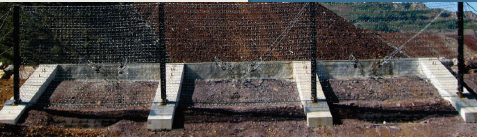
An example of a tree stem impact on a rockfall catchment fence.
