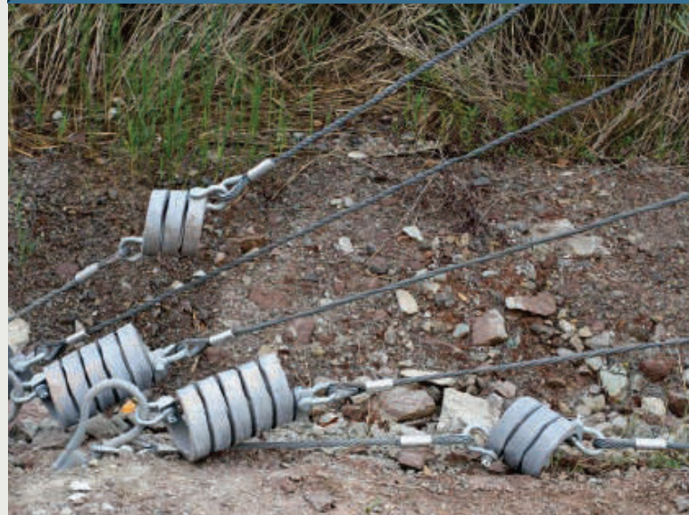
Brake elements are only found at the extremities of a system, directly at anchor points. All brake elements are connected with shackles to the ropes and can be easily changed. In this example, brake elements consist of large steel coils that unwind during impact.
