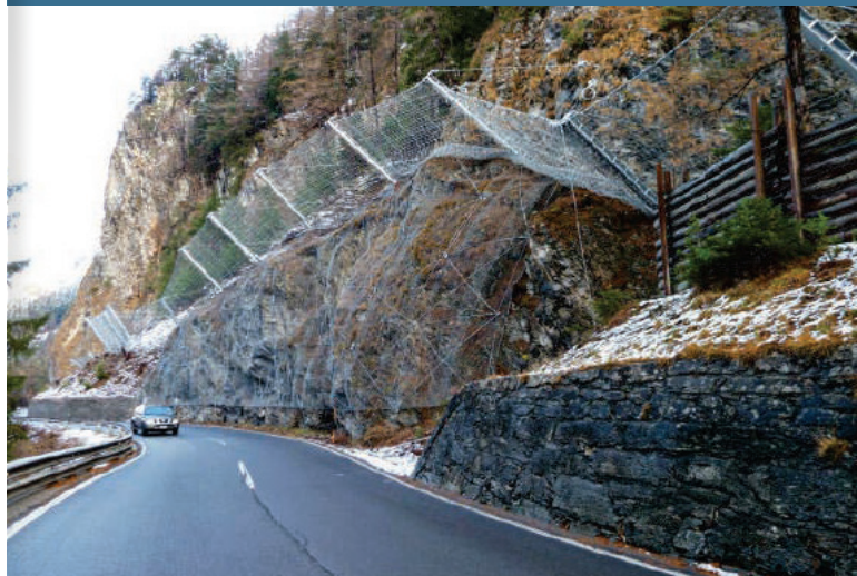
Due to their light weight and minimal foundation requirements, hinged systems are suitable for installation in even the most difficult terrain, including on vertical walls.
