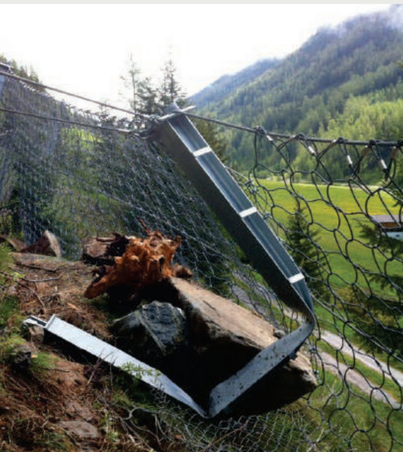
Two examples of hinged rockfall catchment fences impacted at and surrounding a post. These posts are robust and can withstand direct impacts without compromising the systems integrity.
