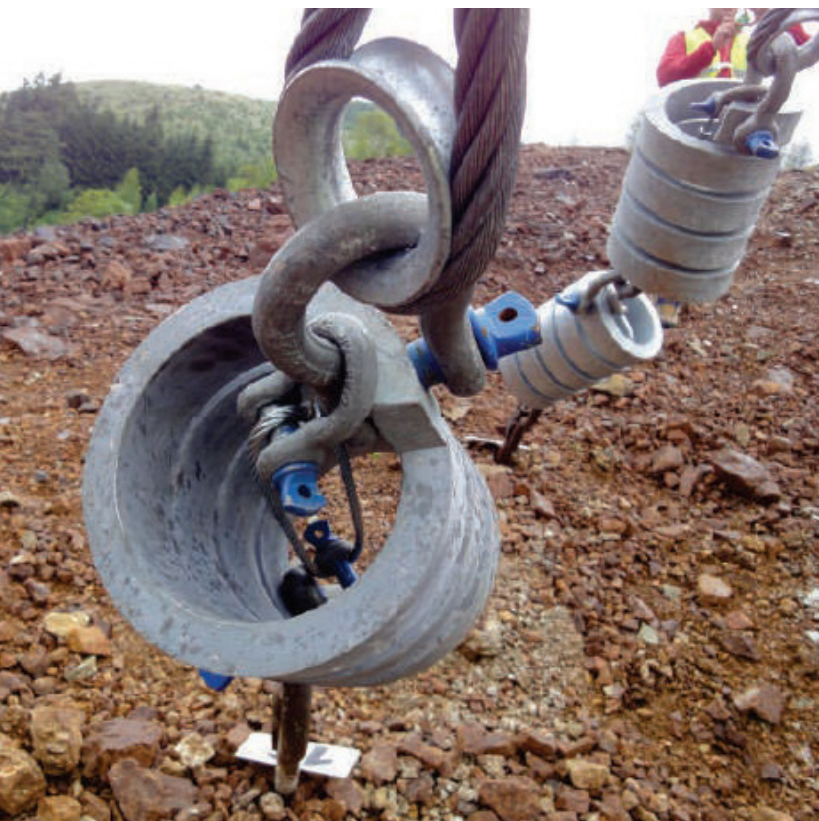
Several adaptations are made to a standard catchment fence to reduce maintenance such as the brake locks pictured above.
