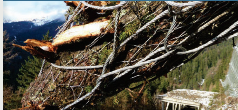
An example of a tree stem impact on a rockfall catchment fence.
