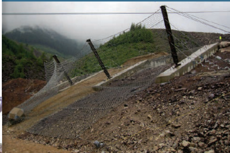
During the impact, the majority of the energy is absorbed during the initial contact with the upper section of the structure, but the projectile is allowed to progress through the system to the bottom portion of the net.
