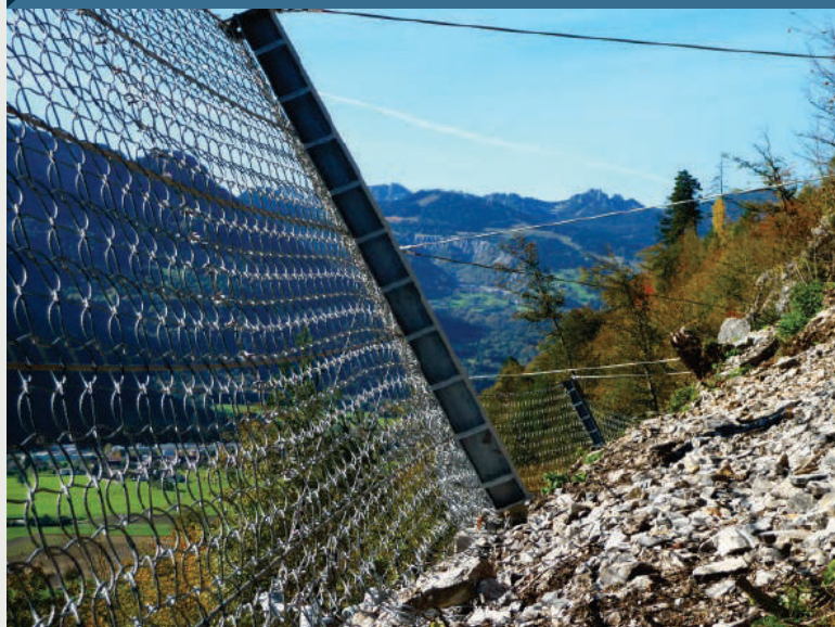
Catchment fences with a hinged connection between the post and base plate require upslope anchors and retaining ropes. As such, large energies can be accommodated while minimizing forces on the foundation of the post.
