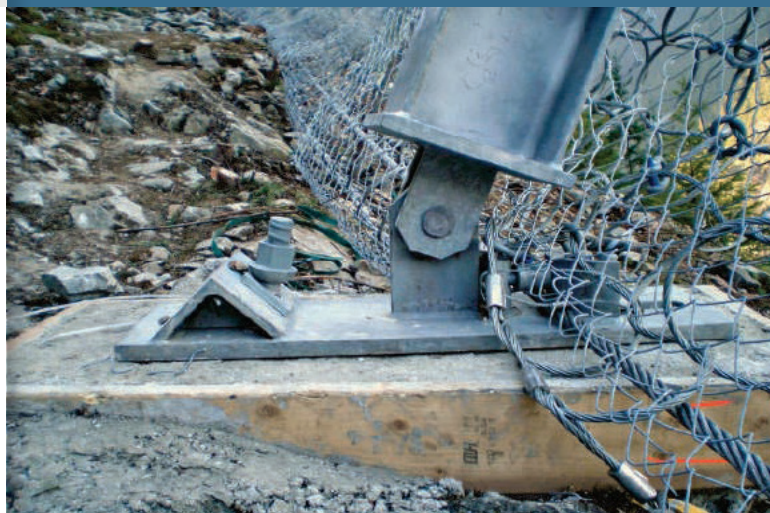
Anchorage for base plates consist of one tension anchor and one compression anchor for ease of installation. Concrete foundations are not necessary though there is full support of the base plate. As such, sometimes small pads are used when in soils.
